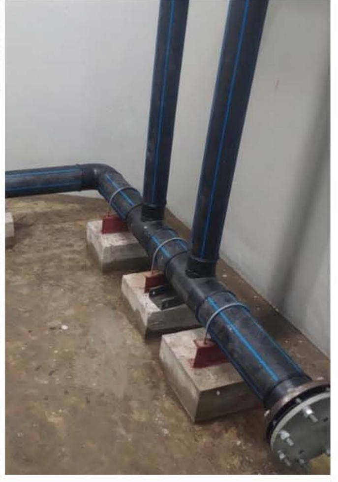
To improve the reliability and quality of the water distribution system at Zone B, we have replaced the old water pipe with new metallic water distribution pipes (HDPE Pipe) this month.
